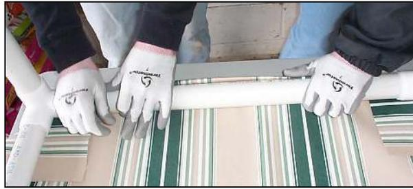
**6** Take one side of cloth, make 2 one-half inch-ish folds. Wrap cloth around pipe. Cloth should hit the center of the pvc on the bottom side of the frame
