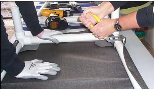
**9** Screw one screw to the opposite side of the frame, then use channel locks to tighten frame. This will tighten the cloth. **IMPORTANT:** Do not use channel locks on top of cloth, it will tear it. Wedge channel locks under cloth to tighten. Tighten so cloth is taught, then screw in rest of screws on that side. Follow the same procedure for the remaining 2 sides. This really is the most important step. The canvas should snap like a drum!
