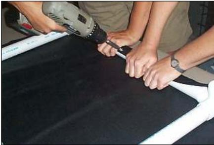
**7** Place one screw in the mid point of the PVC and screw the cloth to the PVC.
